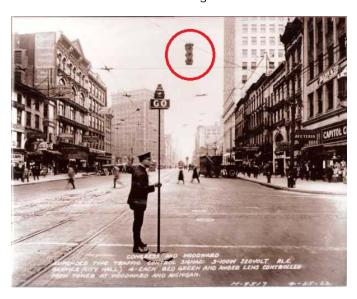
The first of his signals was installed in on the corner of Woodward and Michigan Avenues in Detroit. Within a year, Detroit had installed a total of fifteen of the new lights. The first traffic lights had only four-inch lenses and the shell was wood with a tin cover. An original lamp was presented to Henry Ford's collection of Americana at the Edison Institute, Greenfield Village, in 1938.
